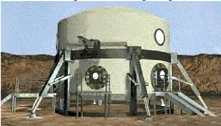
A second such station was erected in southern Utah in 2001.
